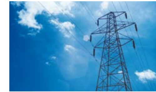
Energy Storage and Distribution
